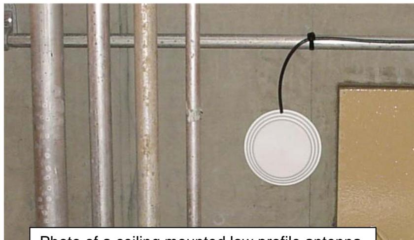
Photo of a ceiling mounted low profile antenna.
